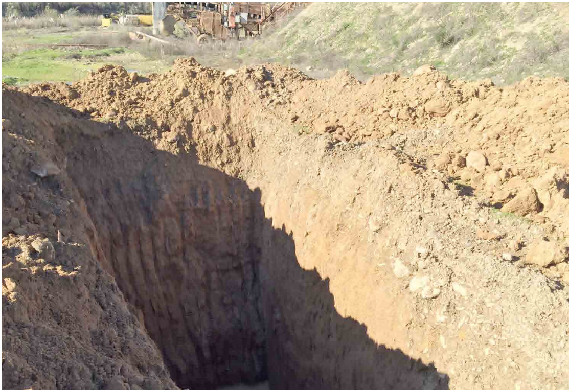
Photo No. 12 Test Pit TP4 in Borrow Area #1 (Clay)
