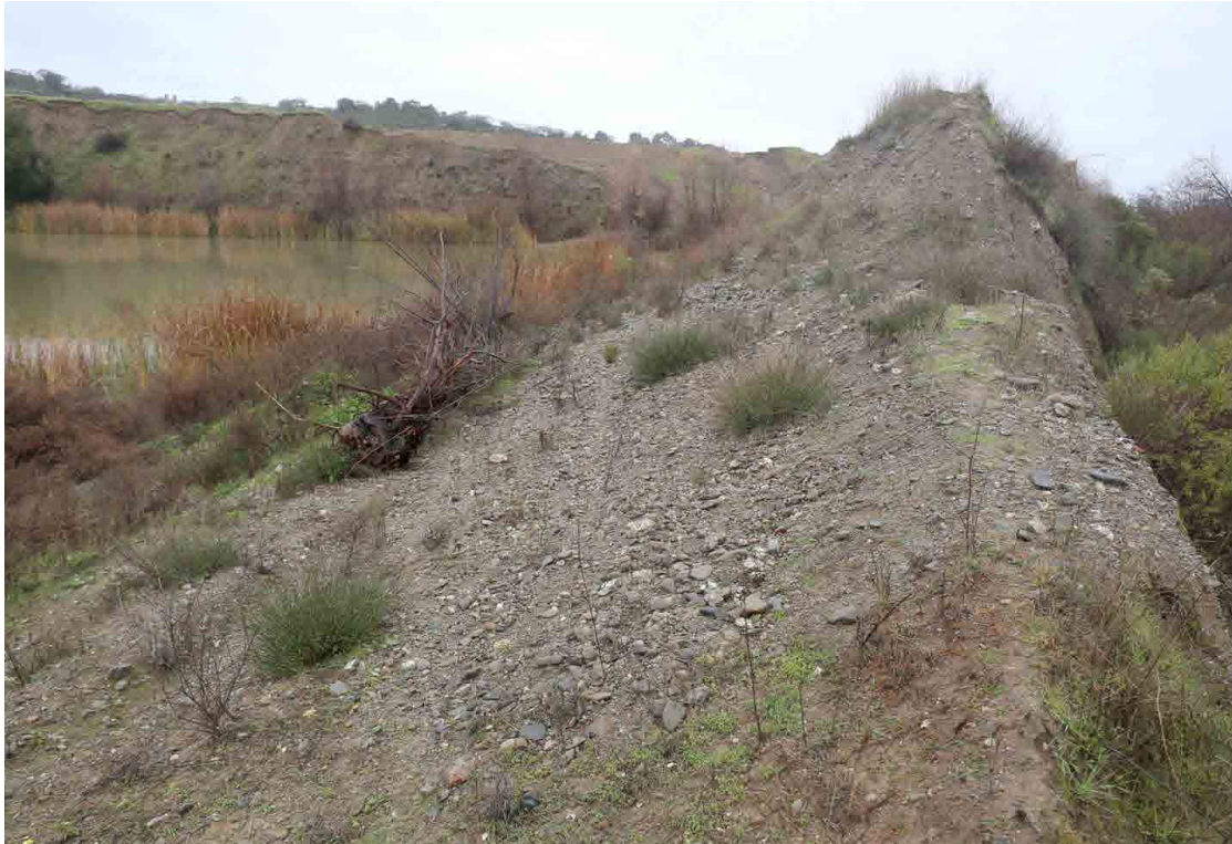
Photo No. 3 Ridge of Quaternary gravel between the Pond west of the Topcon facility and Arroyo del Valle
