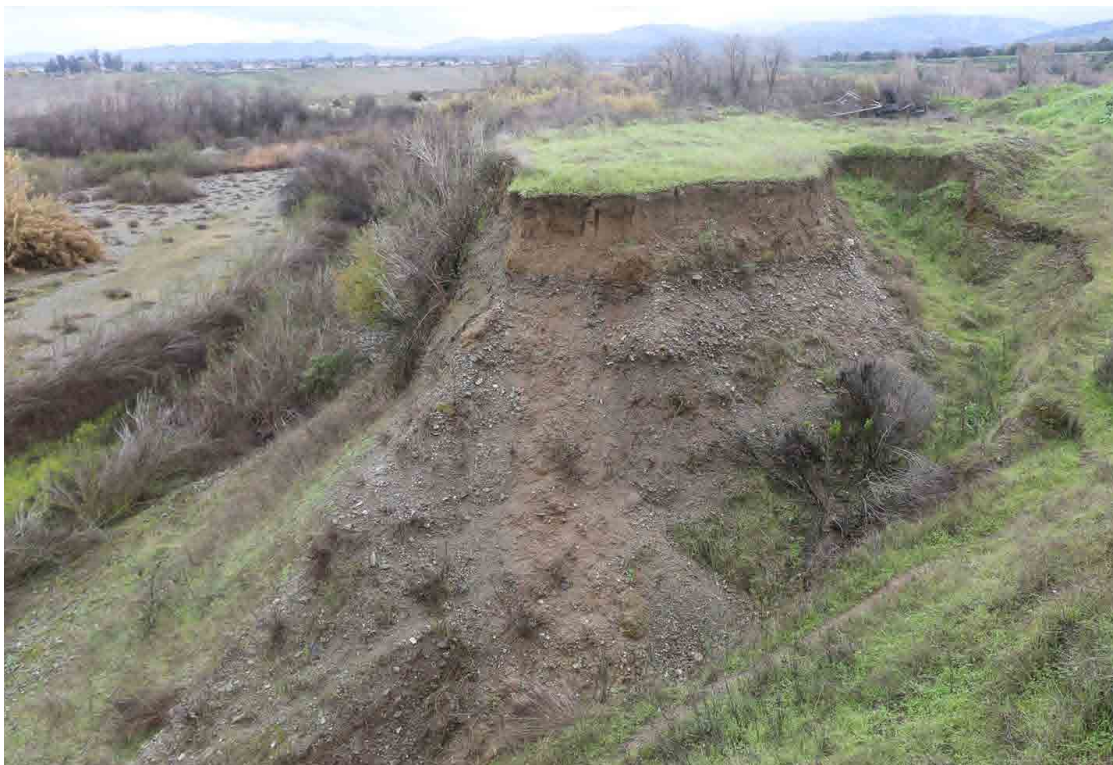
Photo No. 6 Southwest margin of existing Arroyo del Valle west of the Quarry Ponds (looking east)
