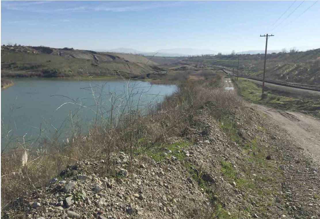
Photo No. 9 Looking southeast at Lake B. Borrow Area #1 (Clay) at far end of the lake
